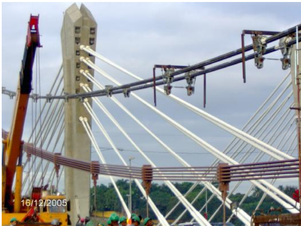
Scaffolding supports on the cable bands
