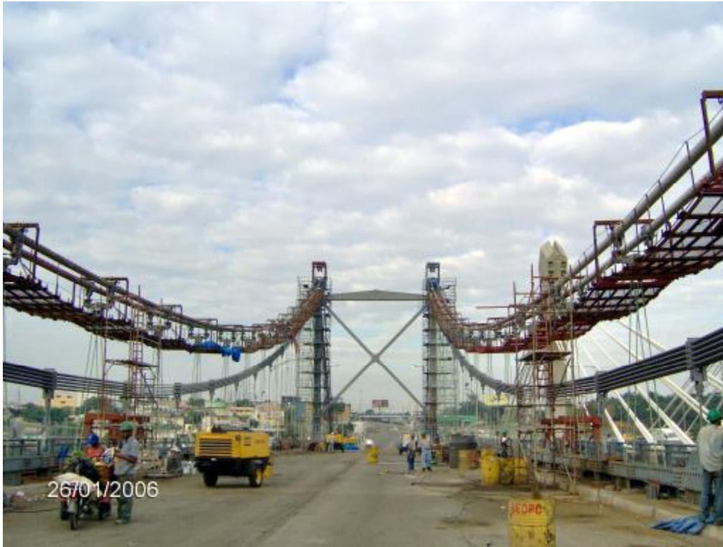
Suspension scaffolding in the central span
