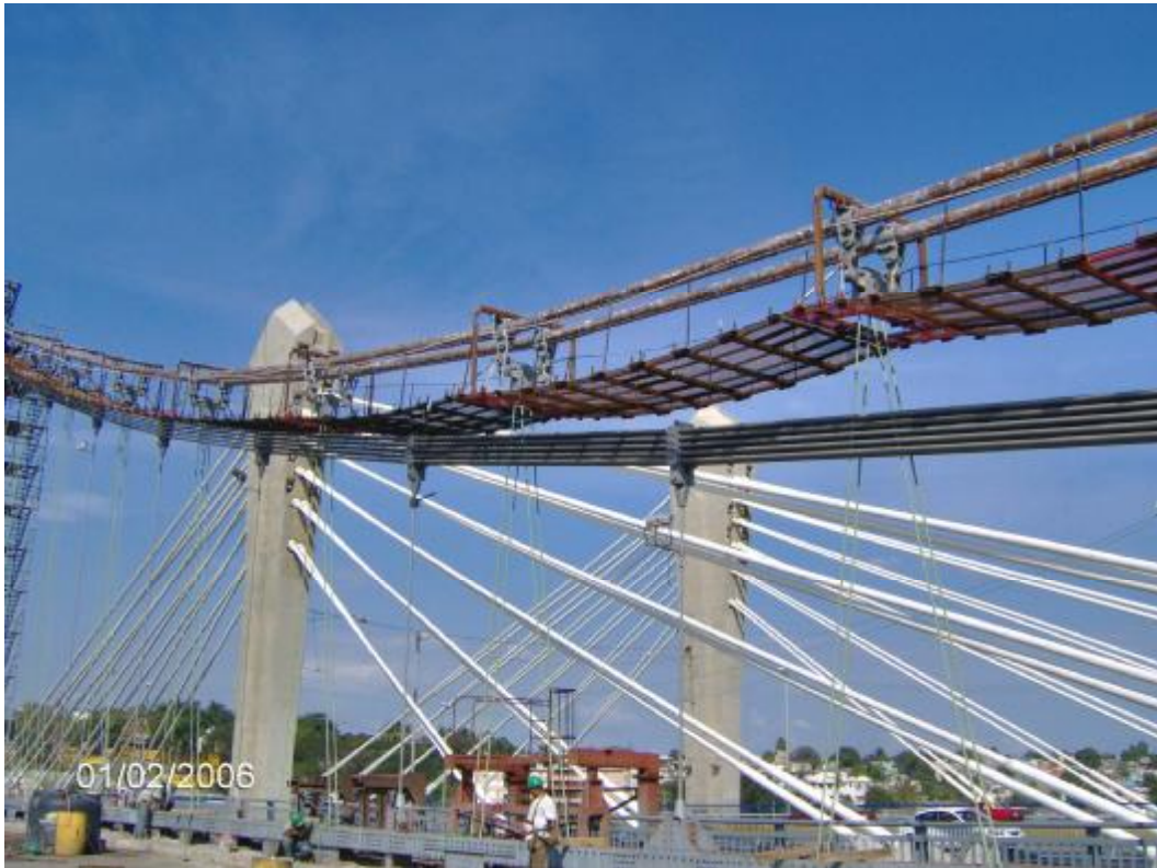
Geometry of the existing and new catenary – hangers in the end quarters of central span are post-tensioned.
