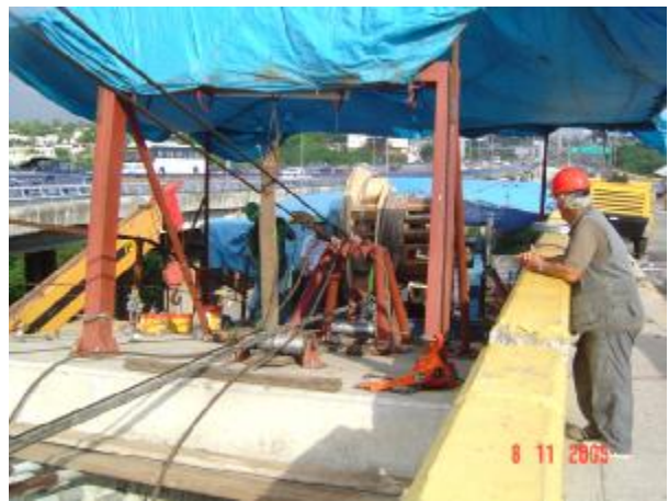
Unreeling of the strand
