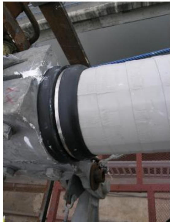
Neoprene sealing ring at the contact with cable clamp
