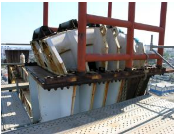
New saddle detail – as found at the beginning of our project
