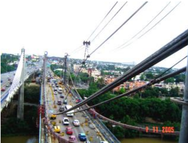
Strand is moving along central span. Bridge is under high traffic
