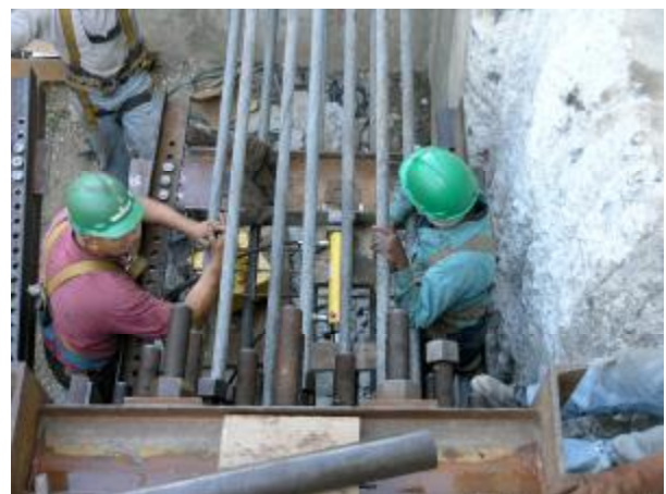
Final adjustment of the strand geometry in the back spans
