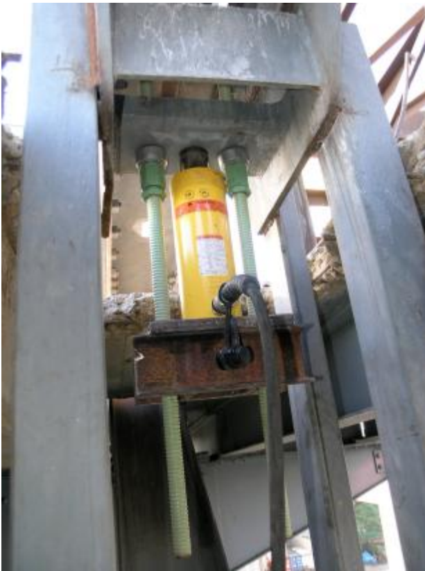
Post-tensioning of the new hangers – 2 ENERPAC 30 tons hollow plunger jacks are installed to pull
