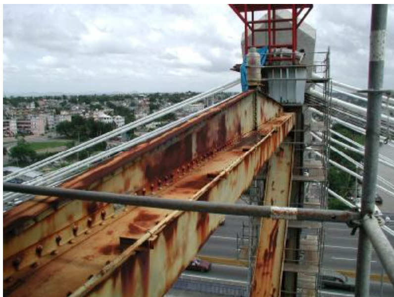
“As-found” corrosion of the bridge steel structure
