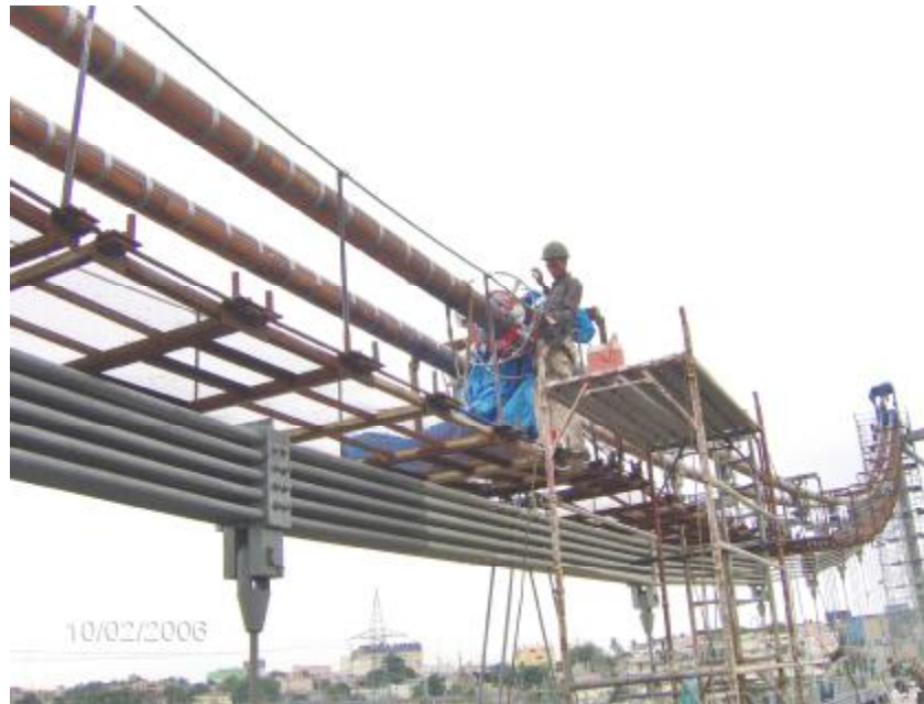
Wrapping of the new cables - CABLEGUARD system
