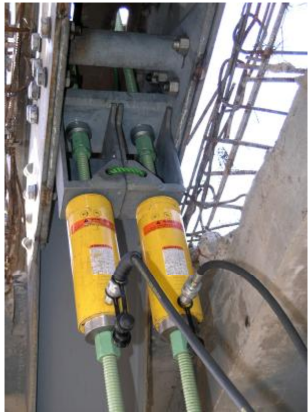
Post-tensioning of the new hangers – ENERPAC 30 tons hollow plunger jack is installed to push
