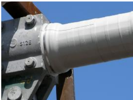
. Contact between cable clamp and CABLEGUARD at the final
