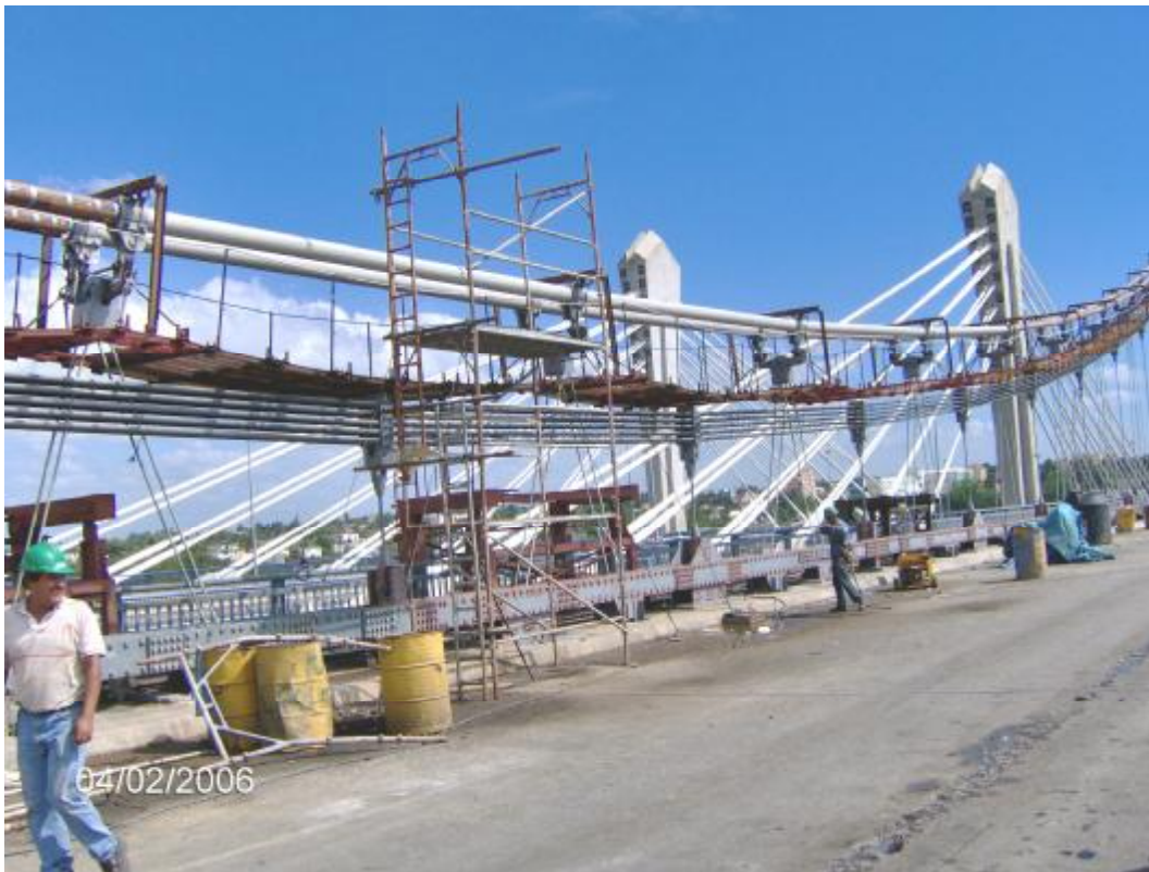
Geometry of the existing and new catenary – almost all hangers are post-tensioned
