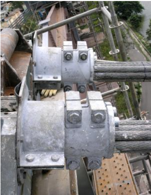
Cable clamps near saddle that should prevent slippage of the strands
