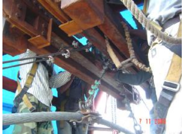
The strand is passing over the tower
