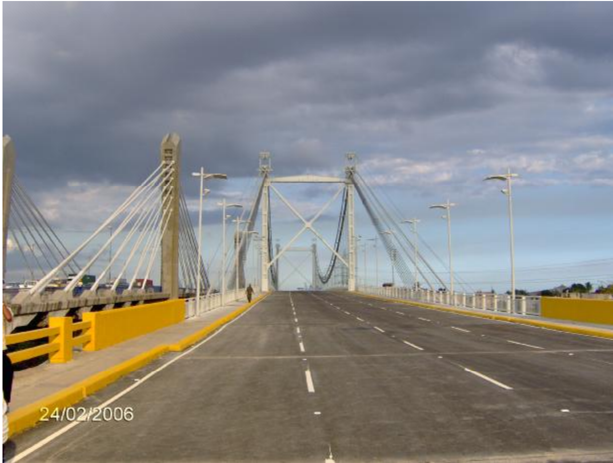
The rehabilitated bridge few minutes before opening.
