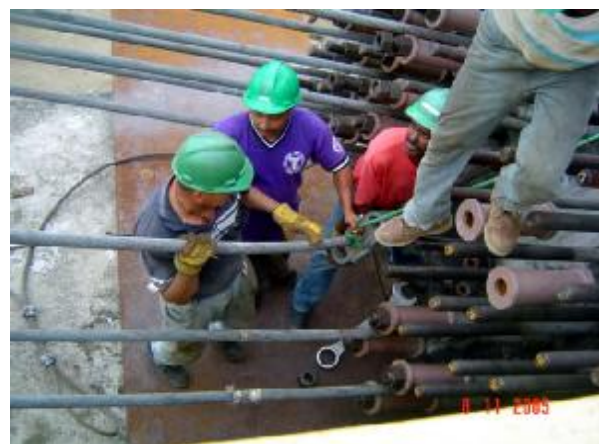
Strand head installation
