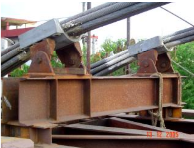
Splay castings near anchor blocks
