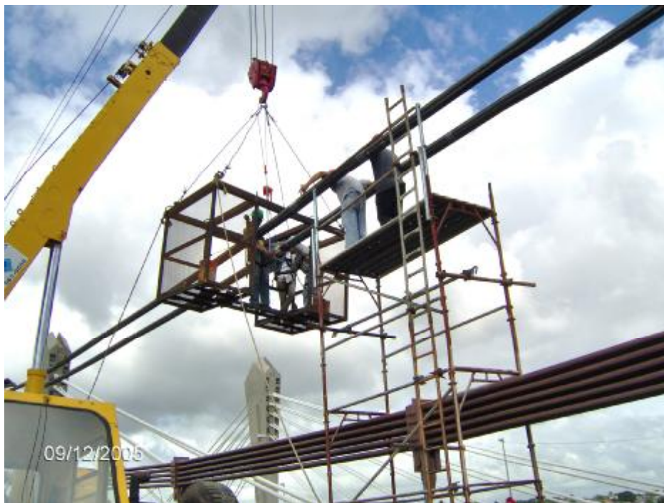
Assembly of the first cable clamp
