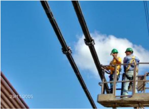
Rollers for fine adjustment of the strand bundle
