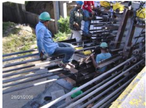
Tensioning of the strands in back spans
