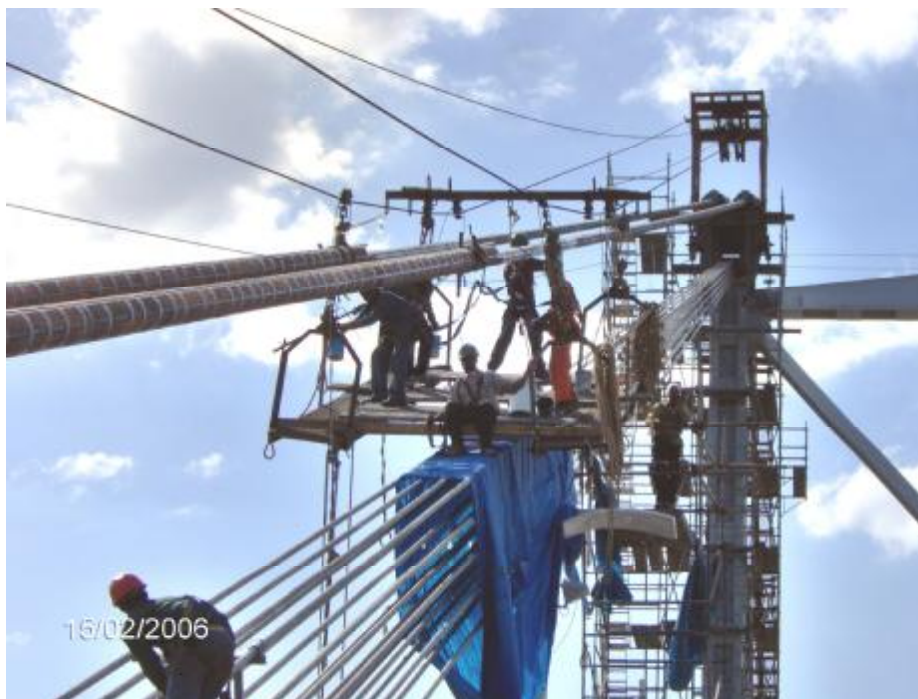
CABLEGUARD installation in the back spans
