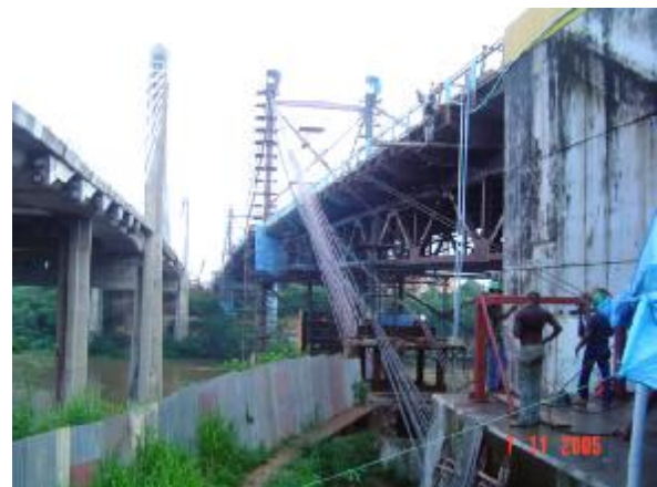
Anchor block on the west – collision of the new strands with existing
