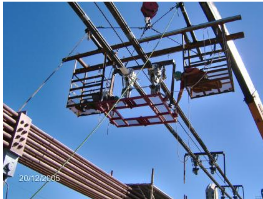
Assembly of the scaffolding platforms
