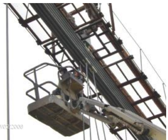
Assembly of the new hangers and protection of the existing strands in the contact with hangers
