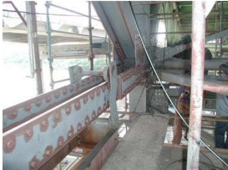
Truss chords are strengthened; steel sandblasted and first paint layer is applied
